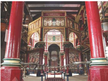
The Crossness Pumping Station, designed by Sir Joseph Bazalgette and opened in 1865.
