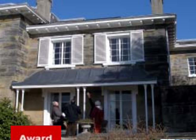
Restoration of the canopy at 8, Calverley Park. (left)
