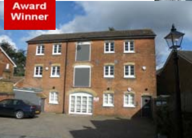
Conversion of warehouse to design studios, Culverden Square. (left)
