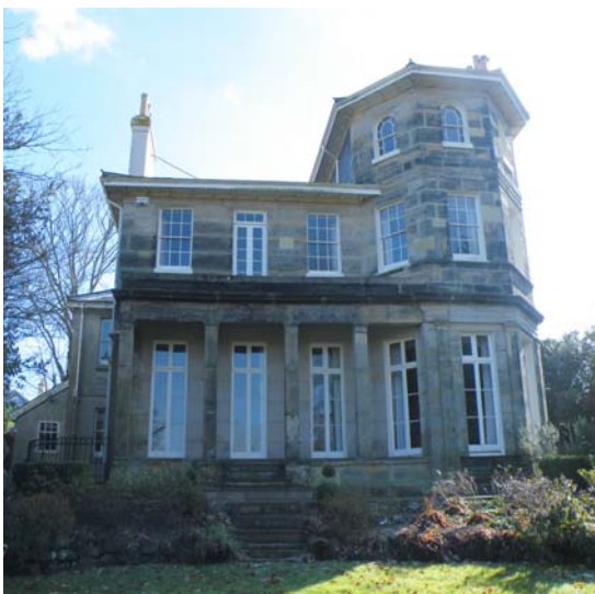
18 Calverley Park before work started.
