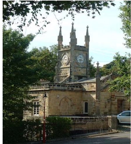
Clock House, by James Burton, c 1828
